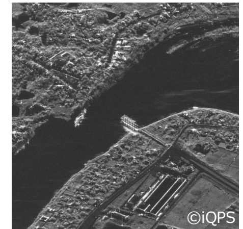
September 2024, Image acquired at Typhoon Damage in Vietnam (Phon Chau Bridge Collapse Section)
